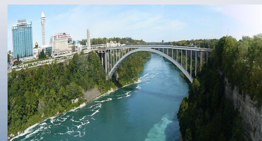
Rainbow Bridge coated with zinc using thermal spray process
